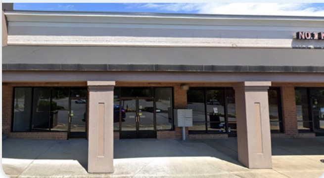
SPACE F - VACANT 1,050 SF
